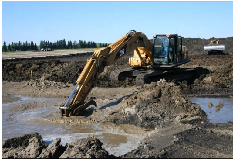
Kyjo Resources Ltd. 00/05-03-041-25W4/0 Bailing rainwater out of excavation May 26, 2012
