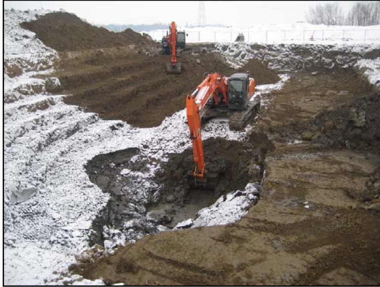
Legal Oil & Gas Ltd. 00/14-29-052-25W4/0 Excavation in City of Edmonton February 6, 2012
