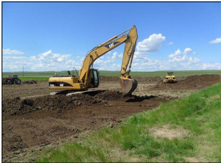
Legacy Petroleum Ltd. 00/16-35-011-02W4/0 Stripping topsoil June 21, 2012
