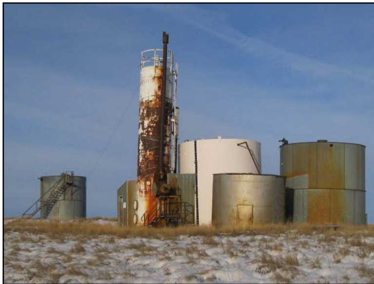
Sarg Oils Ltd 00/12-09-001-17W4/0 well site Storage tanks February 14, 2013
