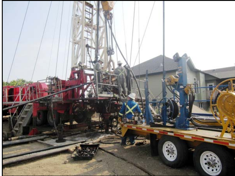
CB Pak Inc 00/04-17-013-06W4/0 Remedial repairs September 24, 2012
