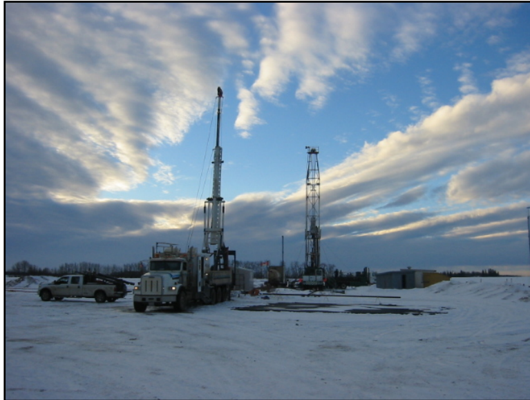
Slate Energy Inc. D0/03-34-055-24W4/0 Service rig during abandonment operations January 18, 2013
